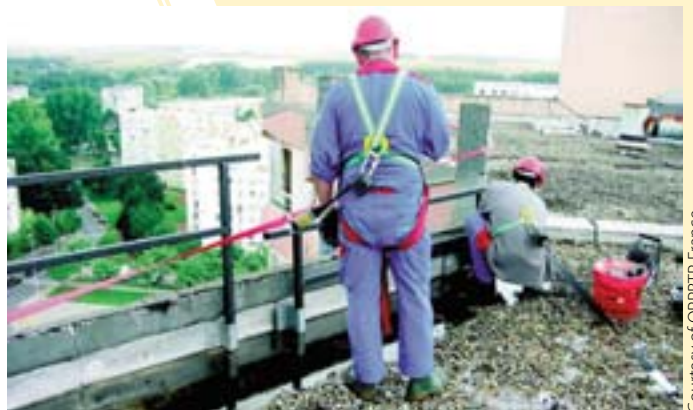
Courtesy of OPPBTP, France
